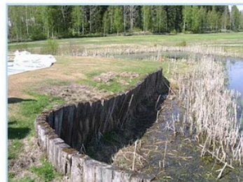
The timber wall is collapsing badly so it would be better to replace it with a steep grass bank
